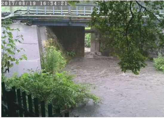
Flood countermeasures in Sawatari River
