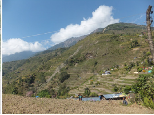
Extraction of slope disaster areas in Nepal
